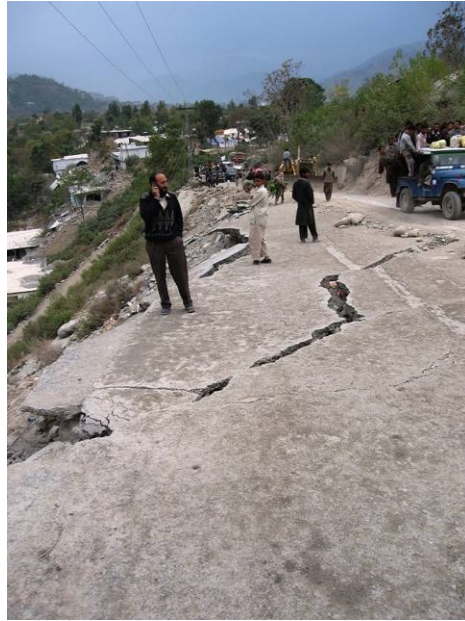
Figure 5.9 Cracked roadway due to land-sliding, north of Muzaffarabad.
