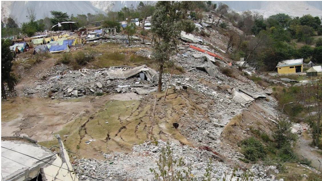
Figure 5.3 Loss of bearing and complete collapse due to land-sliding and ground slumping long a hill edge, north of Muzaffarabad. Notice the ground cracks.
