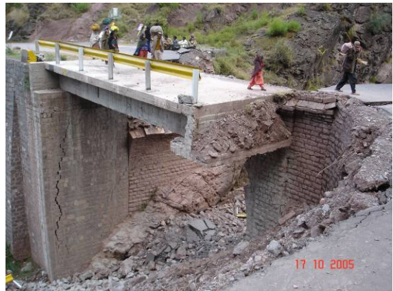
Figure 4.16 Failure of Bridge abutments.
