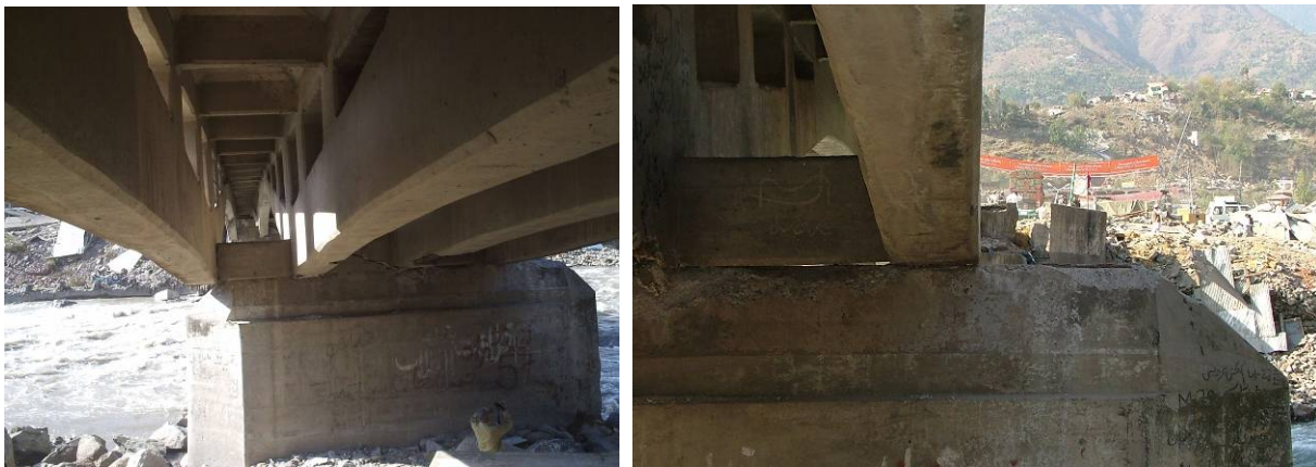
Figure 4.13 (a, b). Balakot bridge that lacked lateral constraint leading to sliding on its bearing supports.
