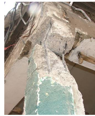
(c) Failure of Beam-column joint
