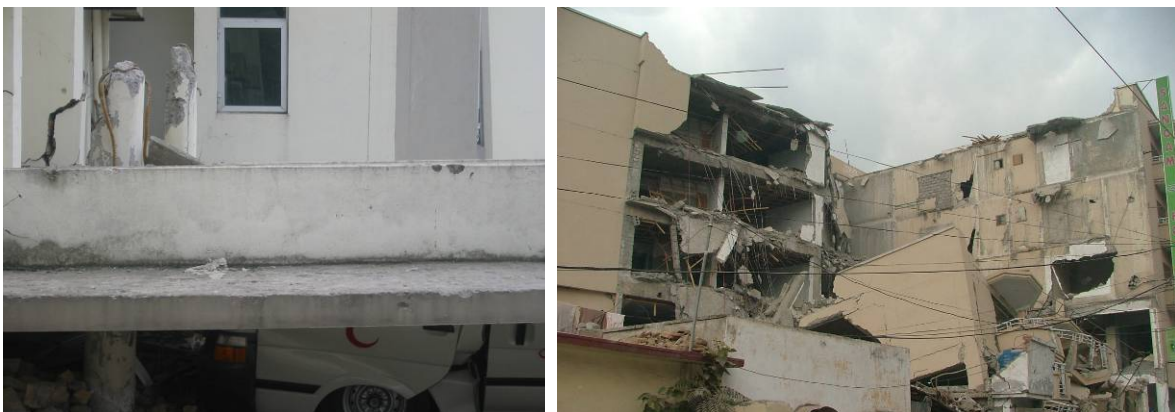
Figure 4.10 (a) Punching failure of the slab in CMH Hospital. (b) Failure of a Hotel Building in Muzaffarabad.
