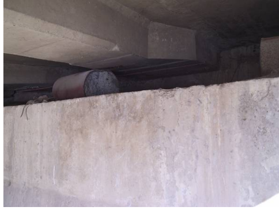
Figure 4.14 (a,b). Left girder is hanging free, remaining girders have just 2 inch bearing left, Balakot Bridge
