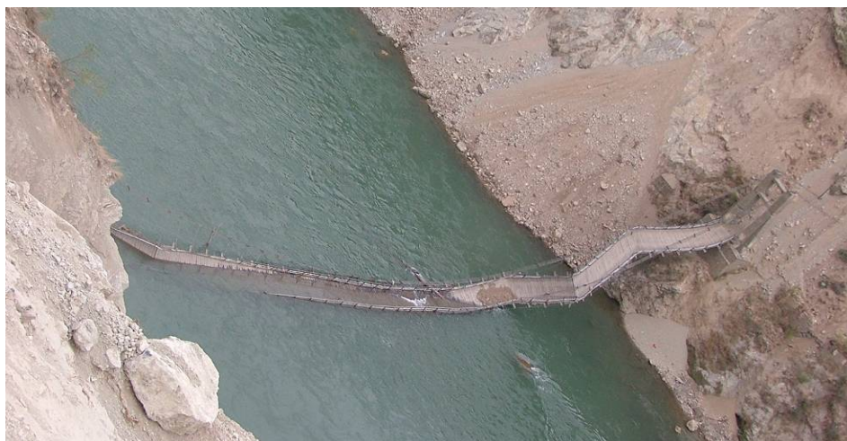
Figure 4.19 Collapsed suspension bridge due to land-sliding, North of Muzaffarabad.
