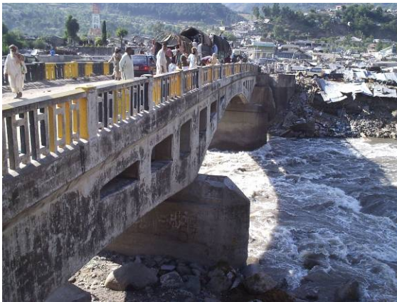
Figure 4.15 Lateral sliding of the Balakot Bridge.
