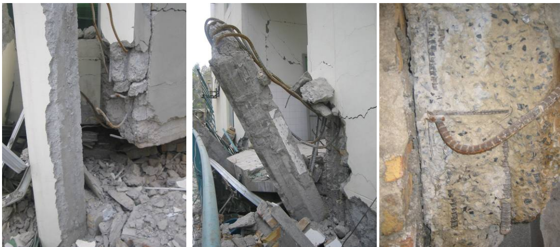
Figure 4.9 (a) Failure of the beam-column connection, (b) failure of the ground floor columns, and (c) the details of the transverse reinforcement, CMH Muzaffarabad
