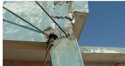
(c) Cold joint and use of undeformed bars
