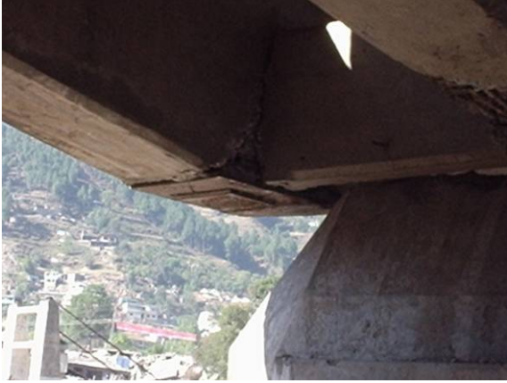
Figure 4.14 (a,b). Left girder is hanging free, remaining girders have just 2 inch bearing left, Balakot Bridge
