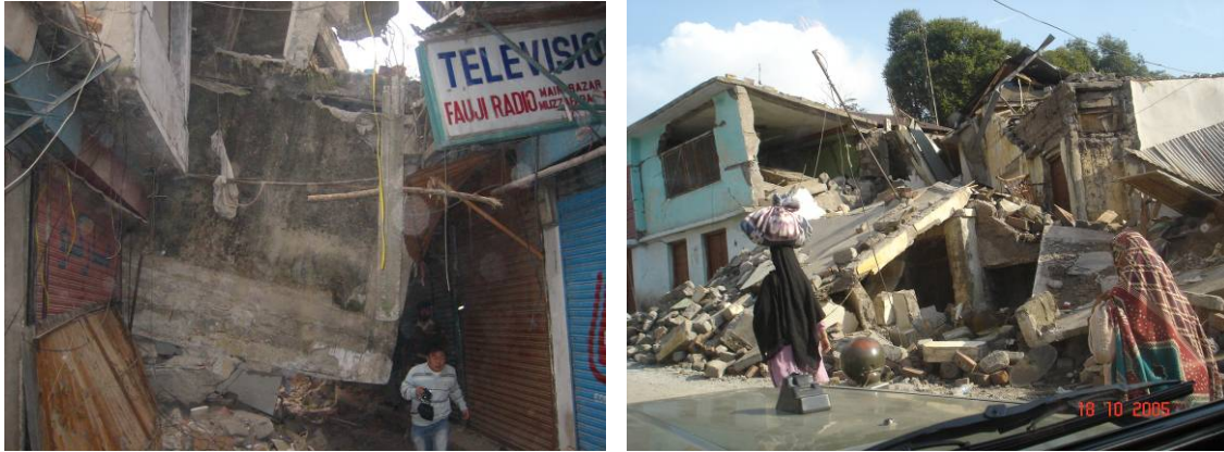
Figure 4.5 Typical old urban and rural housing units made of brick walls and concrete slabs, Muzaffarabad.
