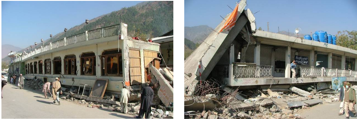
Figure 4.6 Structural failures due to soft story along main street in Balakot
