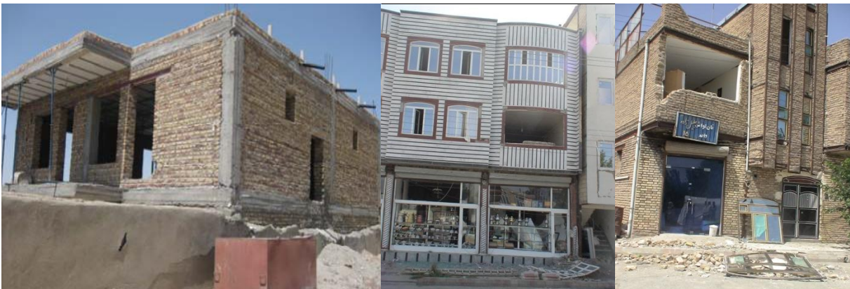
Figure 11. Buildings with minimum code requirement have survived the earthquake (Mehr News Agency; Kalantari-IIIES and Bastami-IIIES)
