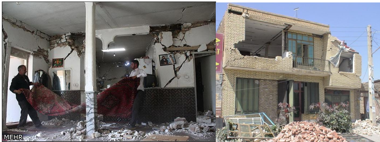
Figure 10. Performance of semi-steel frame buildings in villages (Mehr News Agency and Bastami)
