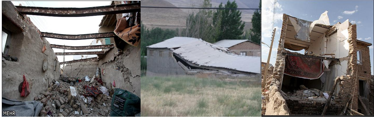
Figure 9. Failure of heavy steel jack-arch and concrete roofs, and walls of UnreinforcedMasonry buildings (Bastami and Mehr News Agency)
