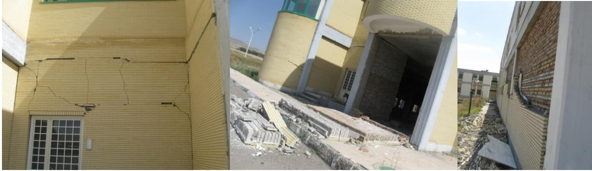
Figure 13. Nonstructural damage to Herris hospital:
