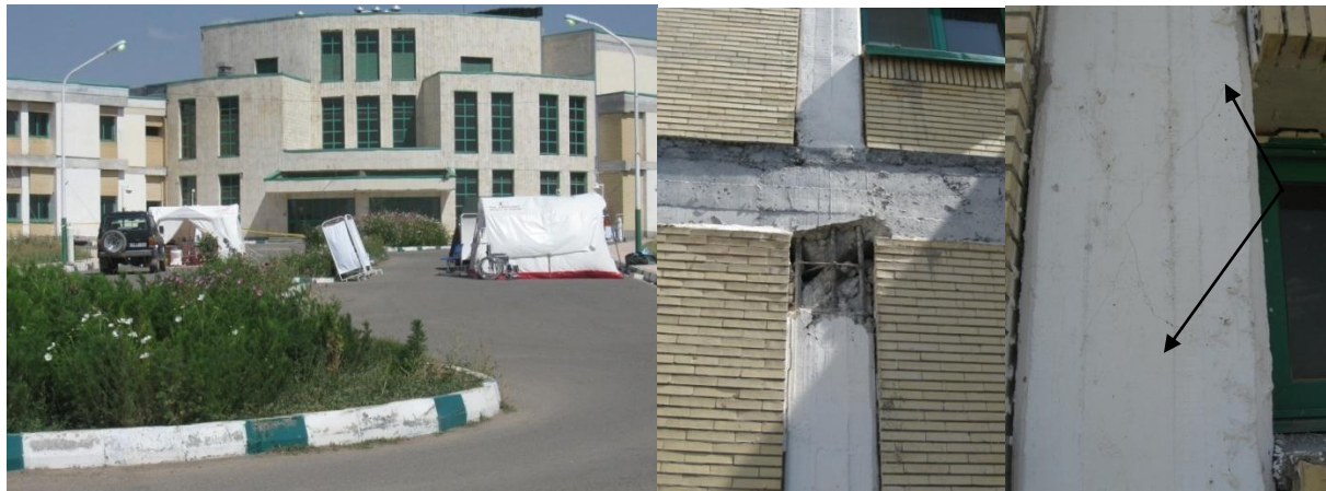
Figure 12. Heriss hospital structural damage to the: Plastic hinges on beam-columns joint and diagonal crack of the column.
