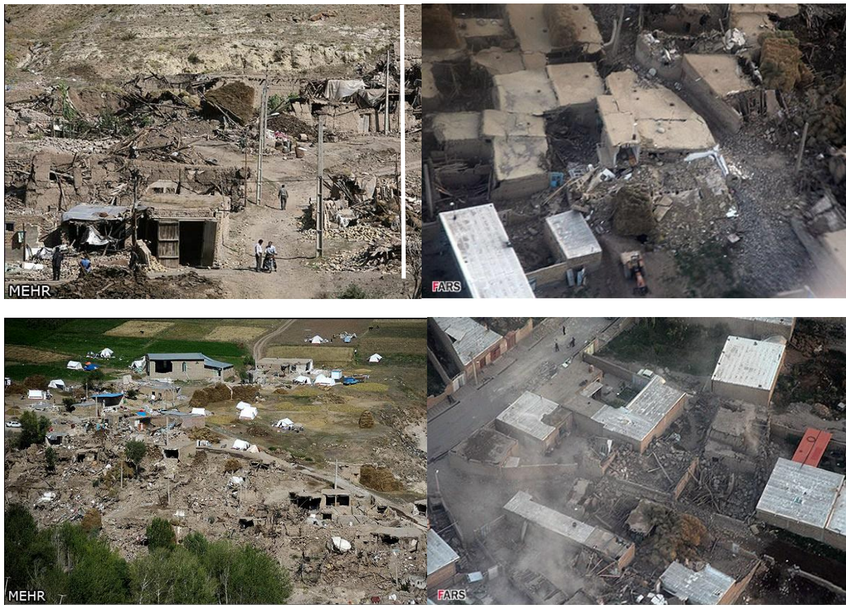
Figure 8. Overall view of the damaged area. It shows that most damages were due the collapse of adobe buildings [Fars News Agencies]
