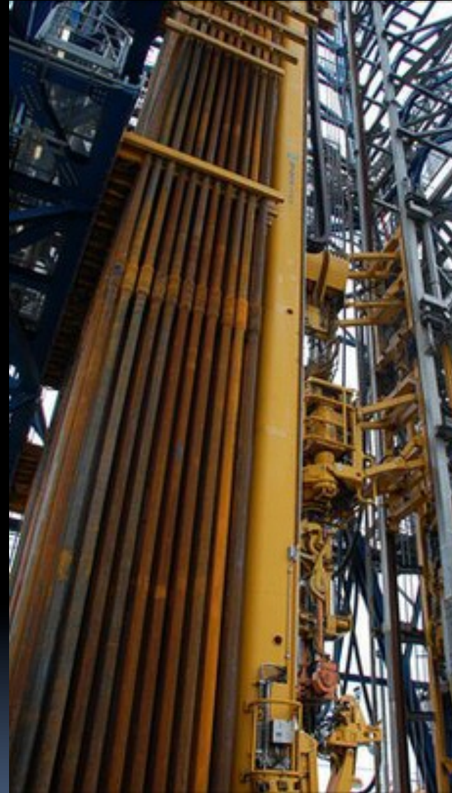
Stands of 36 m pipe
